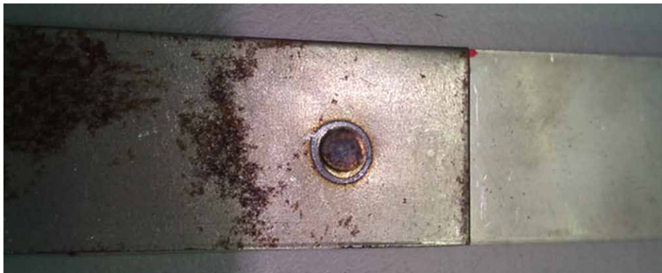
Figure 1. Lap joint of stainless steel and carbon steel sheets
